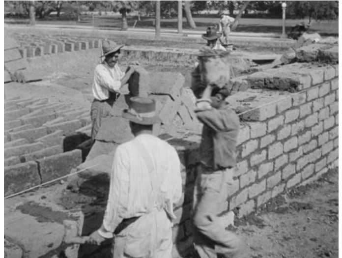
Construction of the walls of Casa de Adobe, 1916.
